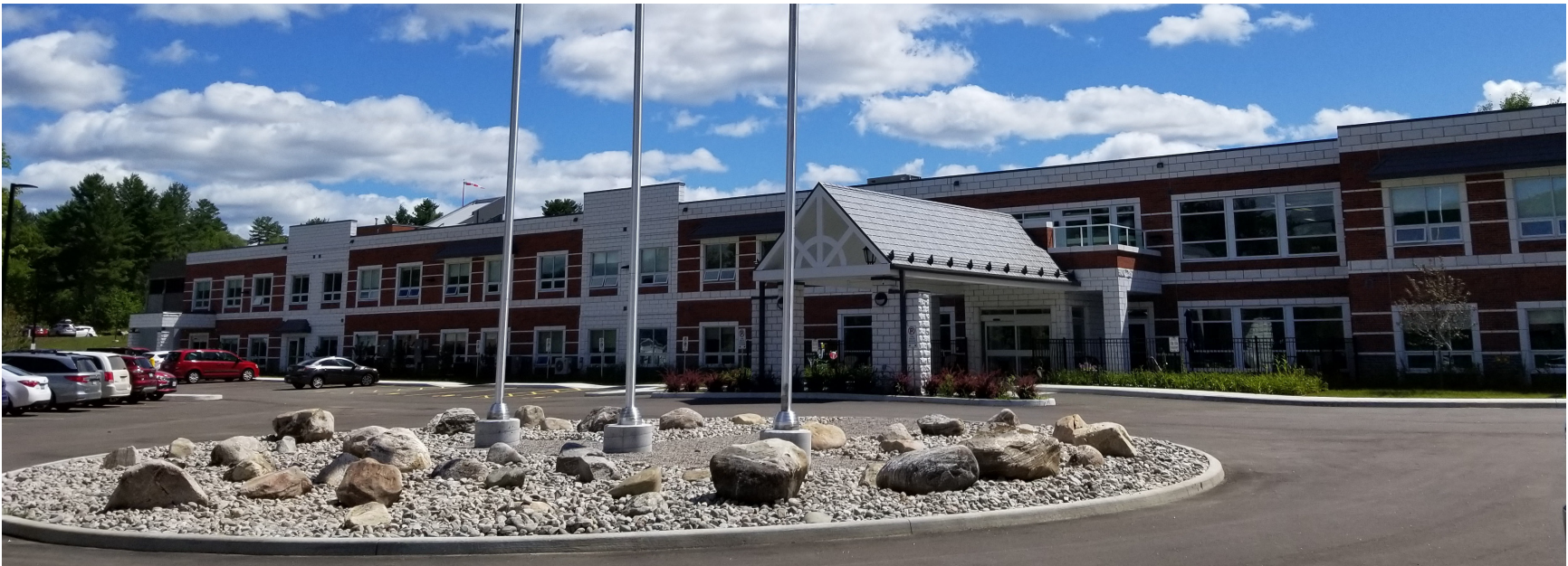
The new Algonquin Nursing Home opened next to the Mattawa Hospital on Turcotte Road in 2019
