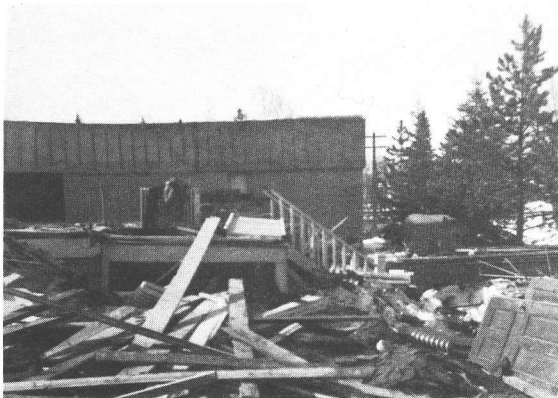
DEMOLITION OF FIRST HOSPITAL, with new hospital in the background — Sixth Avenue looking west
