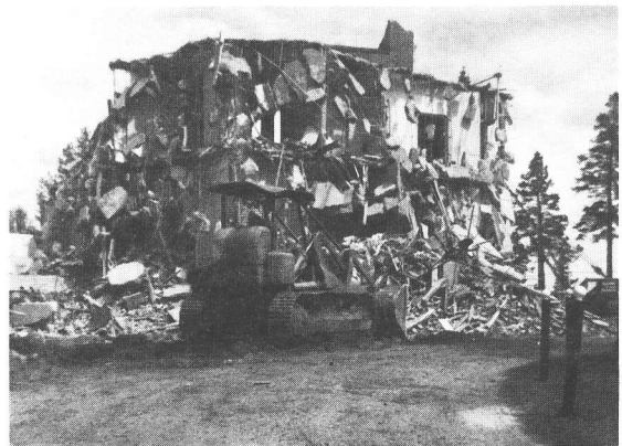
DEMOLITION OF SECOND HOSPITAL, Fifth Avenue, June 1970
