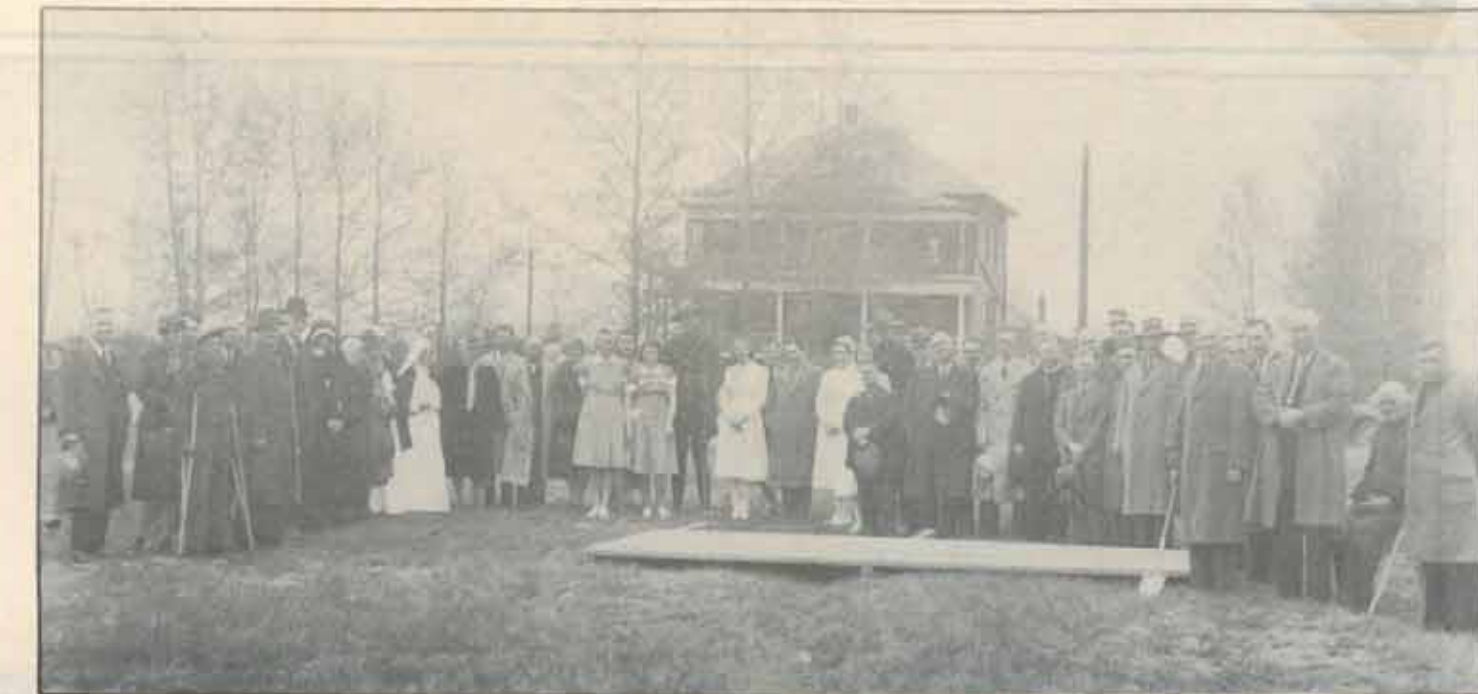
THE SOD TURNING to officially launch the construction of St. Peter's Hospital took place May 14, 1941.
