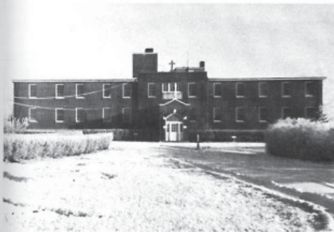
St. Joseph's Hospital showing elevator shaft.
