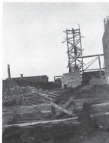
St. Joseph's Hospital construction begins.
