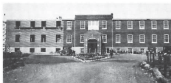
1928 construction of addition
