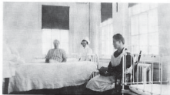
One of the patients' rooms in the hospital
