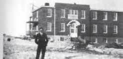
Dr. P.L. Eid on the grounds of the newly constructed St. Joseph's Hospital at Macklin, 1906.
