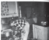
Mr. Toghians and assistant Plumbing Contractor, Fairway Plumbing, Saskatoon.
