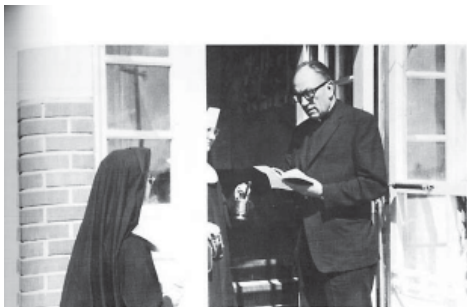
Rev. Joseph Simon, O.M.I., blessing the newly renovated St. Joseph's Hospital.
