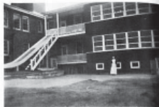
Northwest view of St. Joseph's Hospital showing ramp and fire escape with outdoor balconies. Section of Hospital beyond the balconies and to the right was the sisters' residence. The balconies were removed during the 1964 renovations.
