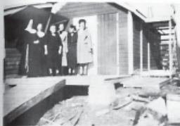
Renovation of employee residence
