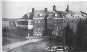
St. Elizabeth Convent and Hospital, as above after the 1919 addition. East side.
