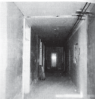
Stage II. Walls and ceilings covered again.
