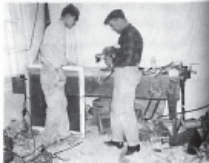
Mr. Peter Fahr, right, and assistant. H.H. Reid construction - Mining contractor.
