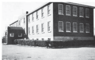
South-West View of Hospital Front Entrance Completed
