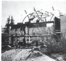
Beams for the chapel are under construction by November.
