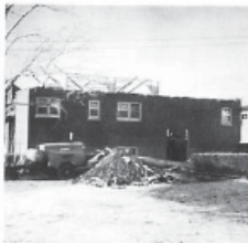
By October the brick walls were under construction.
