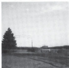
Driveway to front entrance of hospital.
