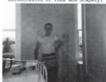
Representative of Hudson Bay Co. Installation of rods and drapery.
