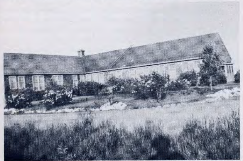
Side View of Airport Hospital
