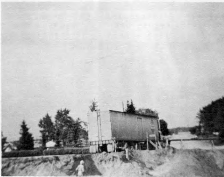
June 4, 1964, First Load of Steel
