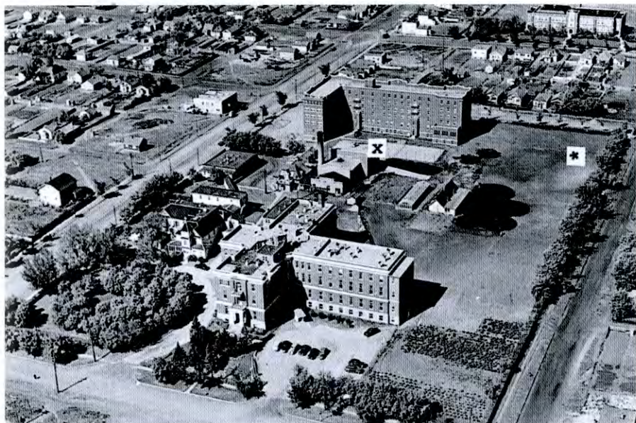
Air-view of hospital grounds (1948) with two locations of boiler room.
