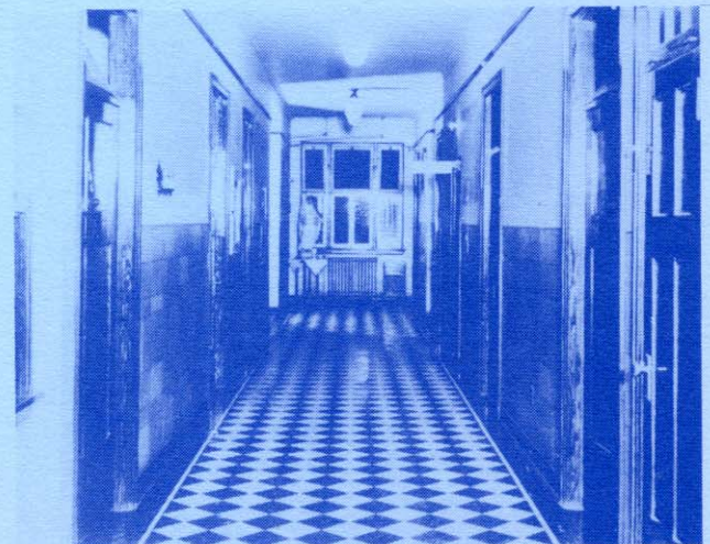
1935 First Floor Hallway
