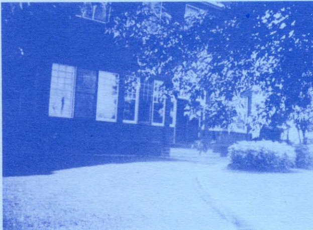
The closed in balcony around the 1934 converted this first floor into a children's pavillion.
