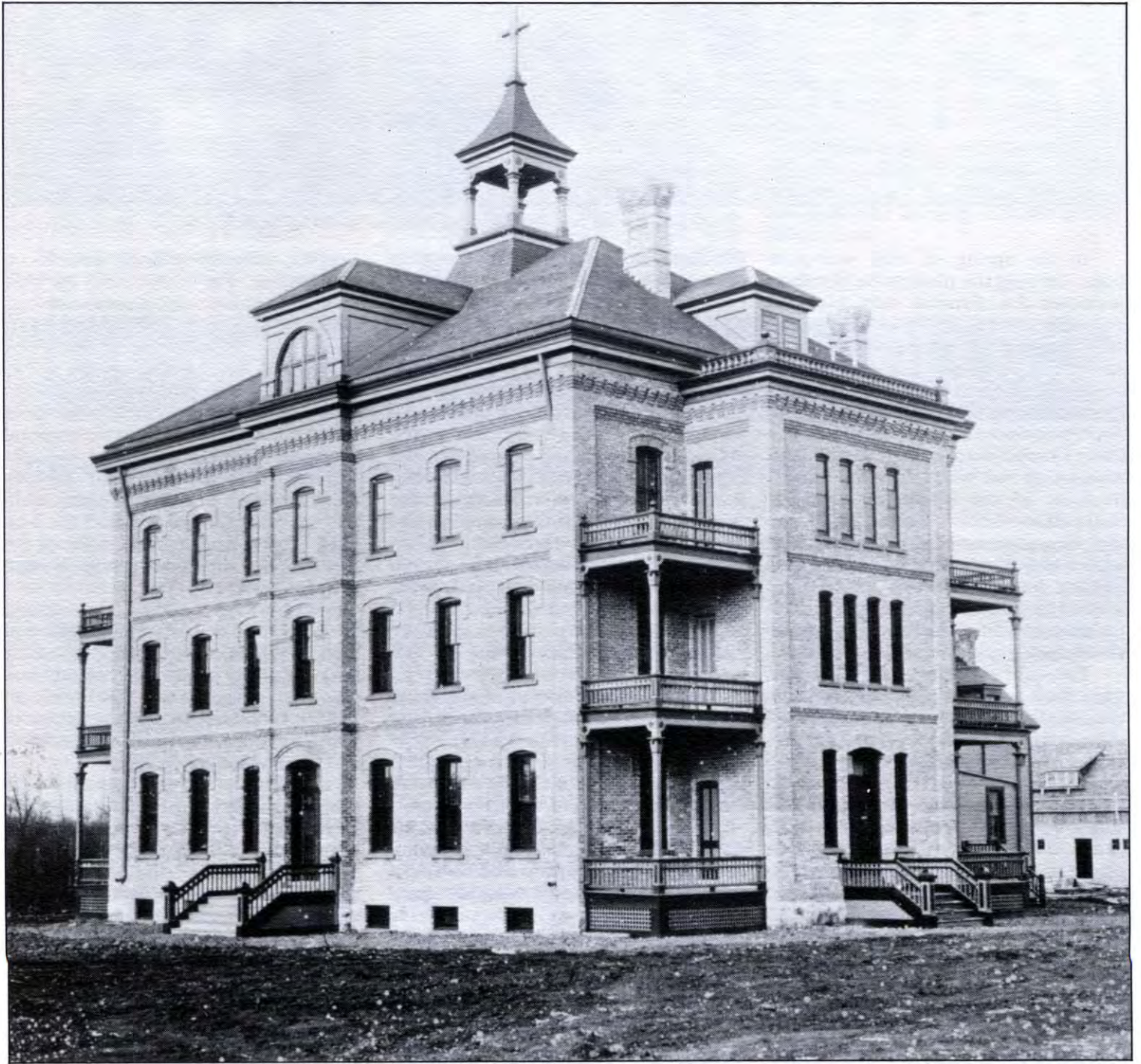
The original Edmonton General Hospital.
