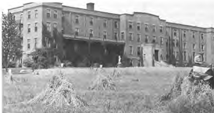
Bethany Motherhouse after 1937 addition.
