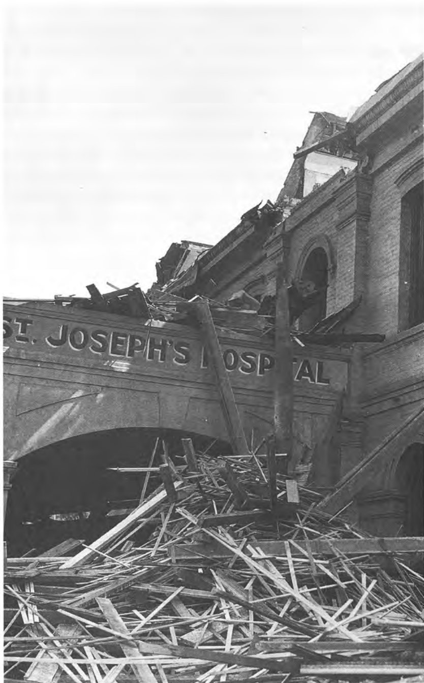
Demolished in 1949, the original 1876 portion of St. Joseph's Hospital had aged to the point of being considered a fire hazard. In its place a new wing of the hospital was built. SSAA P0235
