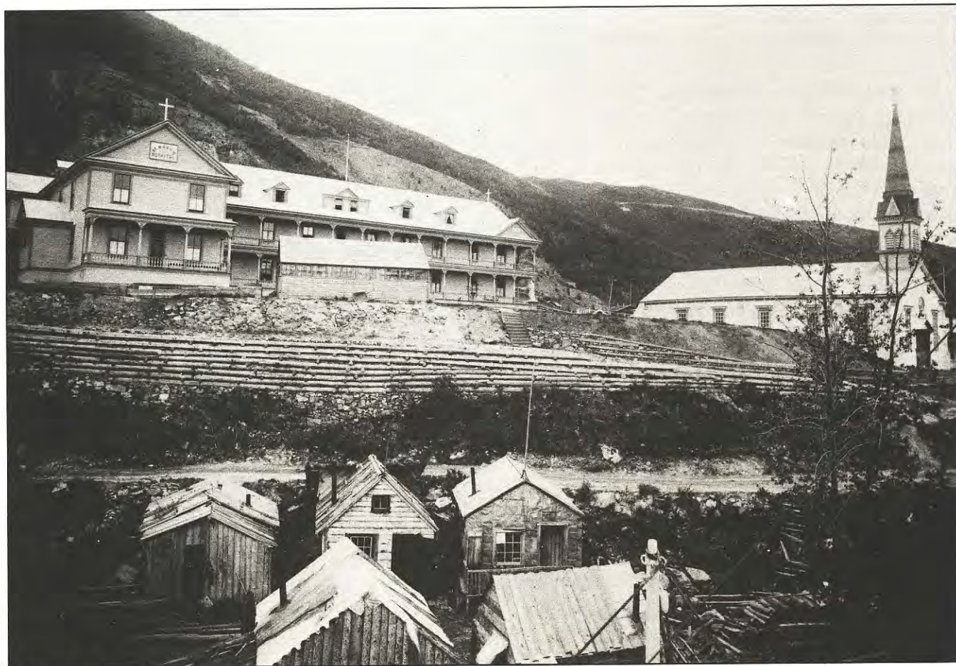
In 1906, the old structures were demolished and the new 3-story hospital was built to serve Dawson and the area. The greenhouse gave a start to flowers and vegetables and was a precious asset to the grounds. Patients looked for signs of greenery as the winter days dragged on. Some of the extensive cribbing necessary at the site shows up well in this post-1909 view. (SMA)
