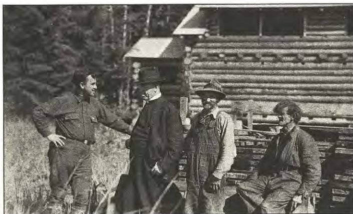
At the Shrine of St. Terese, under construction in the 1930s, concerned enterprisers have a discussion. (l. to r.) Father Bernard Hubbard, S.J., Father William LeVasseur, S.J., Mr. Joe Brown, Mr. Henry Meyer, builder. The log lodge is immediately behind them.
