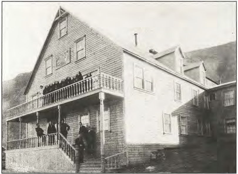
Dormer windows and 2-level balustrade porches are reminiscent of the hospitals in Juneau and Douglas. The similarity is even more striking in the 1906 development. (SMA)
