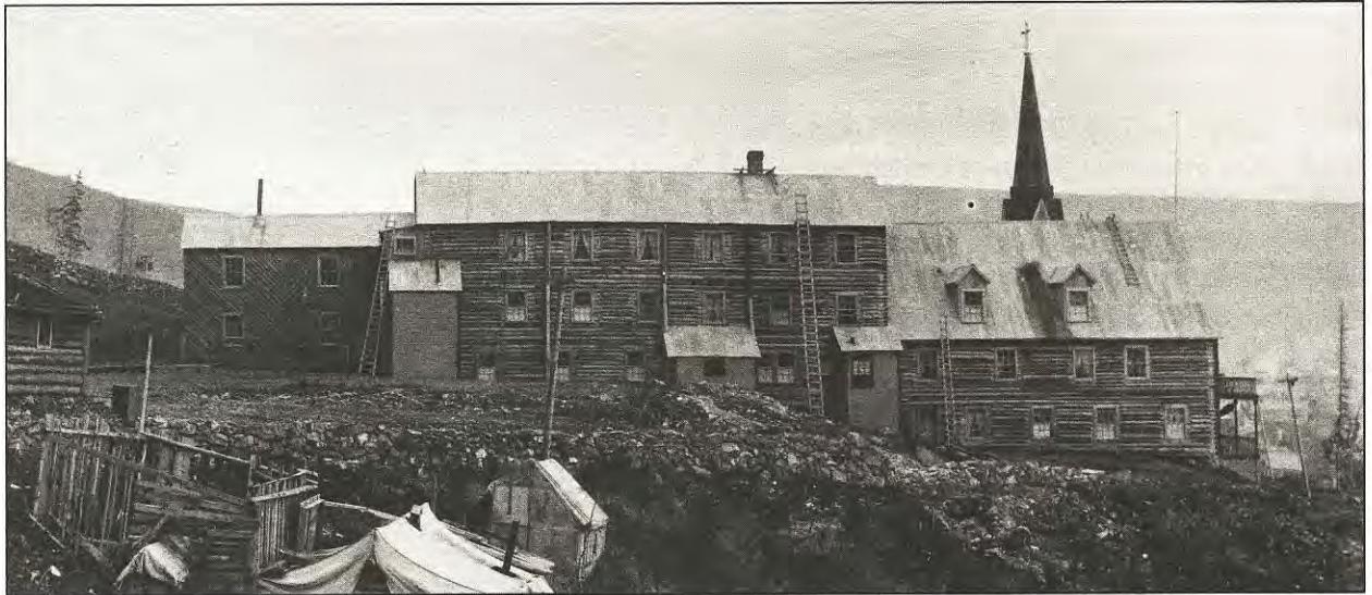
This side view shows additional structures at St. Mary's. (SPA)
