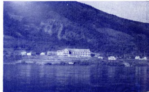
Saint Mary's on the Banks of the Yukon The Jubilee Extension is seen under construction—to the left.
