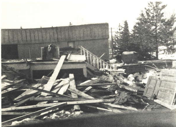
Demolition of first hospital, with new hospital in the background – Sixth Avenue looking west.
