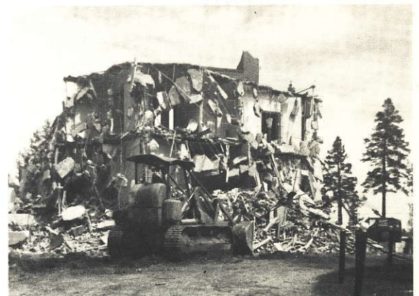
Demolition of second hospital, Fifth Avenue, June 1970.
