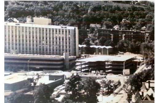
Construction of Parking ramp 2 1986
