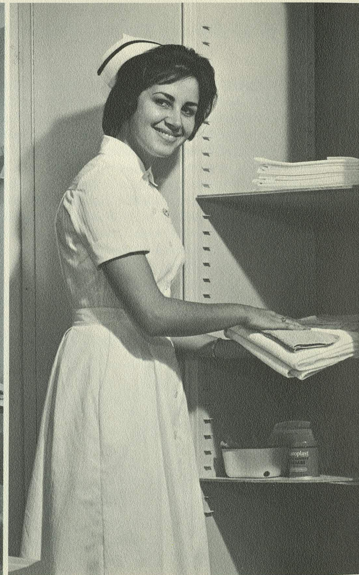
Each room has a built-in nurseserver, with twin compartments—one for clean linens and nursing supplies, and a separate, suction-ventilated compartment for soiled materials and utensils.
