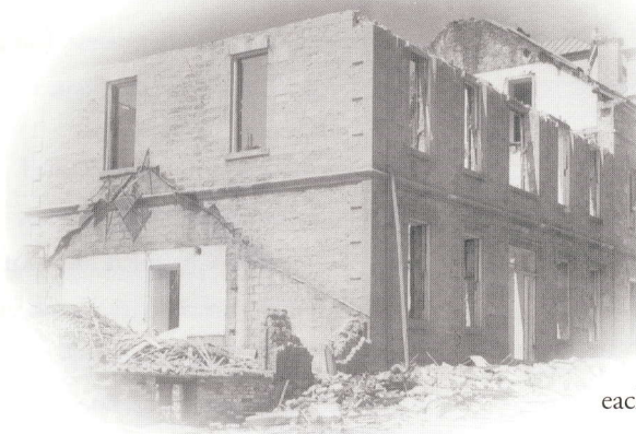
Demolition of the 1862 and 1877 House of Providence – 1959.
