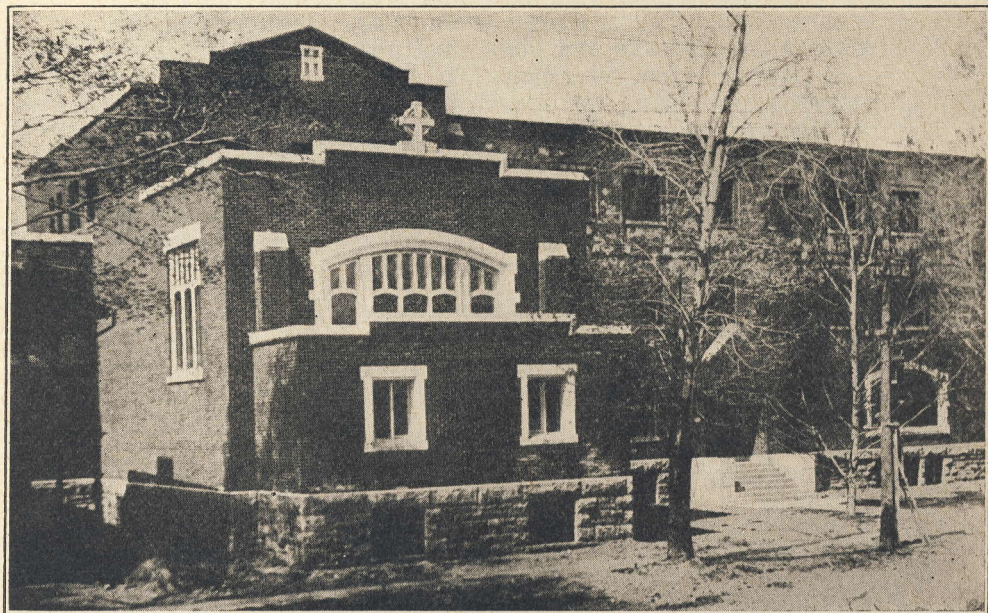
FRONT VIEW OF MONASTERY
