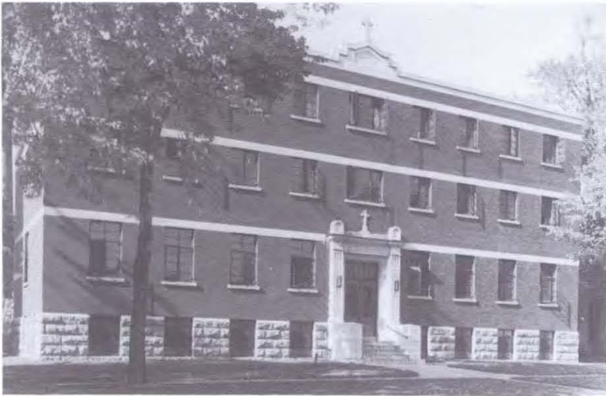
This new building for St. Joseph's School of Nursing and the Nurses' Residence opened on York Street in 1939. It replaced the Greenwood and McTiernan Houses, which had been student residences since the School first opened in 1929.
