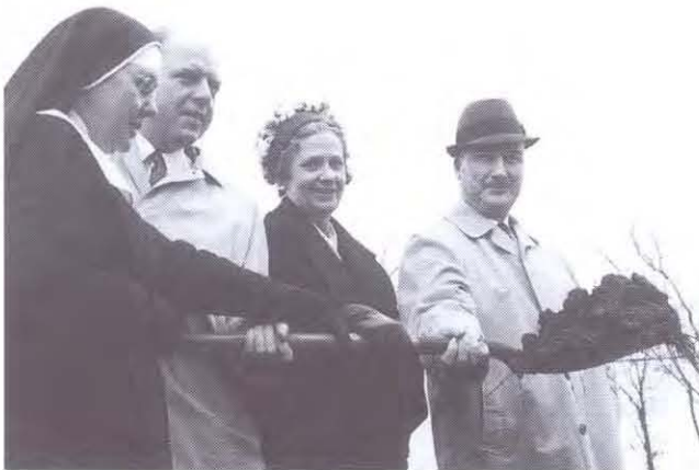
When the sod was turned for the $1.3-million Regional School of Nursing on April 4, 1967, those collaborating represented several institutions. Treasurer of the new school was Sr. Mary Murphy (left), Administrator of Hotel Dieu Hospital. D.A. Robertson, President of the Board of Governors, was also Administrator of Cornwall General Hospital. Mrs. Tatiana Labekovski, School Director, formerly taught at St. Joseph's School of Nursing. At right is Irvin Brown, Vice-President. The Regional School was completed in June 1968. (Photo by Ken Gosling)
