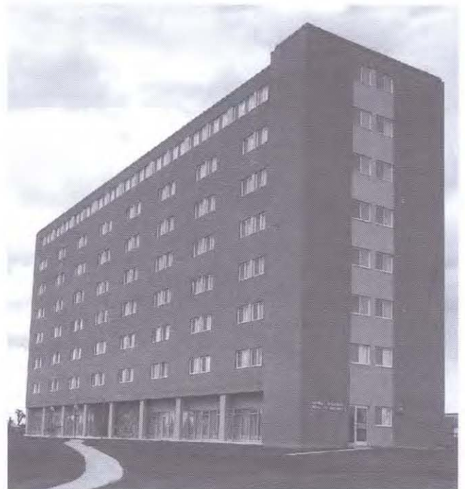
The Regional School of Nursing at the corner of McConnell Ave. and Fourth St. was a nine-storey building with classroom space for 200 students and residence space for 144. (Photo by Ken Gosling)
