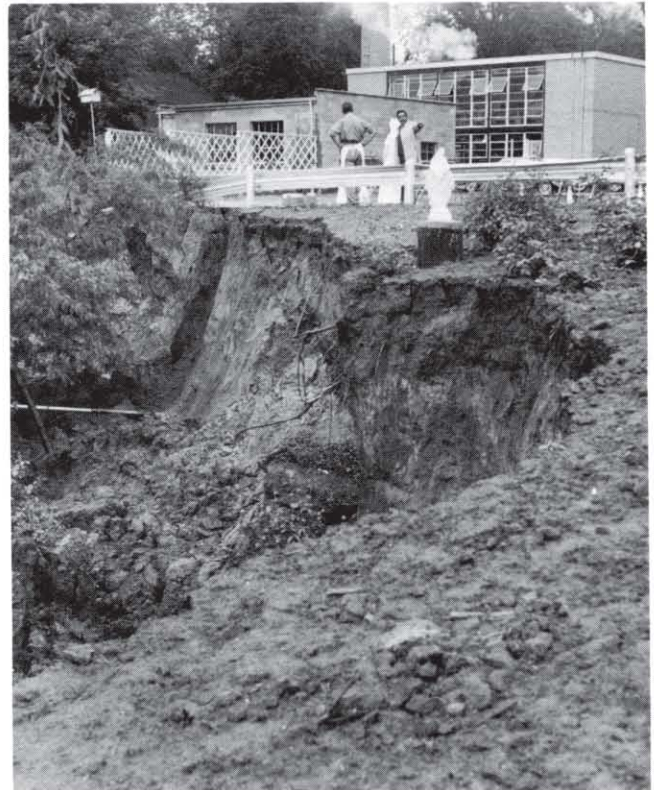
Riverbank erosion — June 8, 1964.
