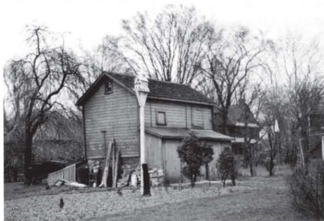
Old barn behind Nurses' Residence where boiler room stands today.
