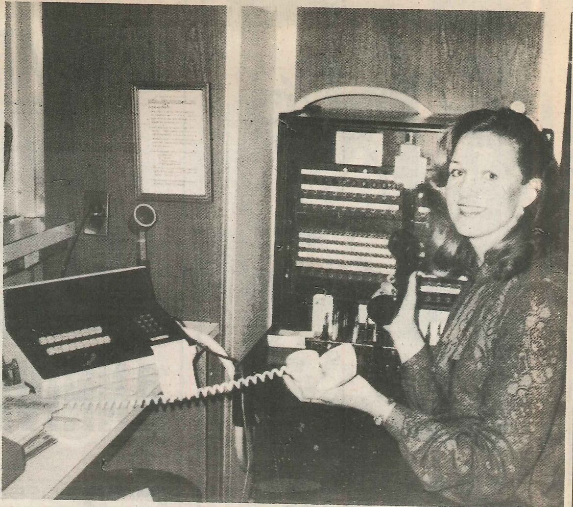
This photo of Yvonne Fournier taken in 1983 shows the difference in equipment on the day the new switchboard was installed.
