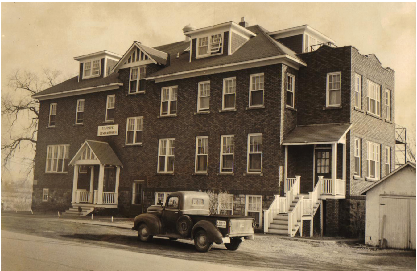
St. Joseph's Hospital, Blind River ~ With cottage roof prior to 1955.
