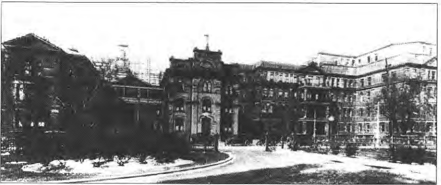
St Michael's Hospital c. 1912. The original hospital is in the middle, the Hugh Ryan wing on the left, and the 1912 addition (the D-wing) on the right. The original exterior walls of the 1912 addition are still doing their work in 1992, housing – among other services – the CV-ICU.
