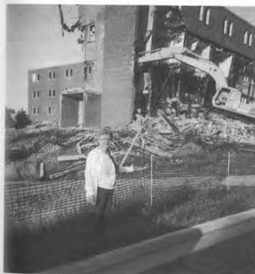
Demolition Ignatius Hall behind St. Rita Hospital 1998.
