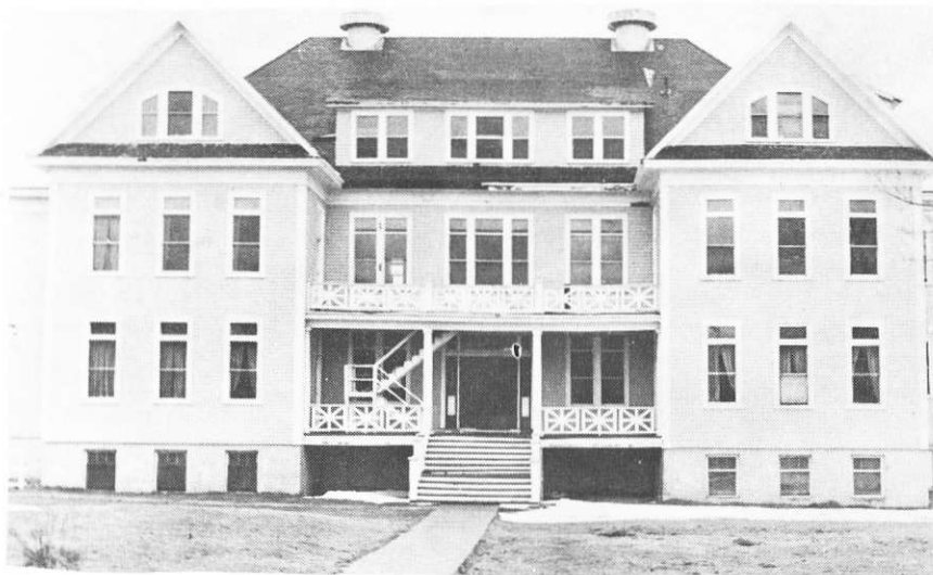
The New Waterford General Hospital was converted in the mid 1960s to become the Miners' Memorial School.
